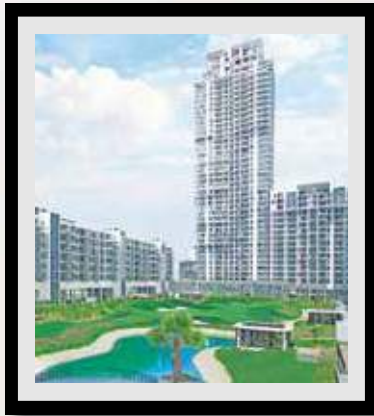
M&M golfestate Fairway GOLF COURSE ROAD EXTENSION SECTOR-65, GURUGRAM
